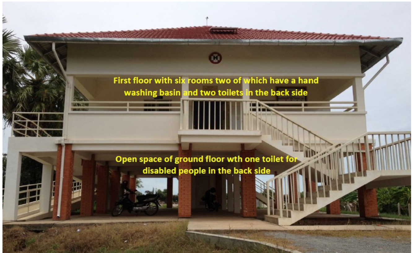
Figure 1: Picture of a health centre of the current design in Cambodia
