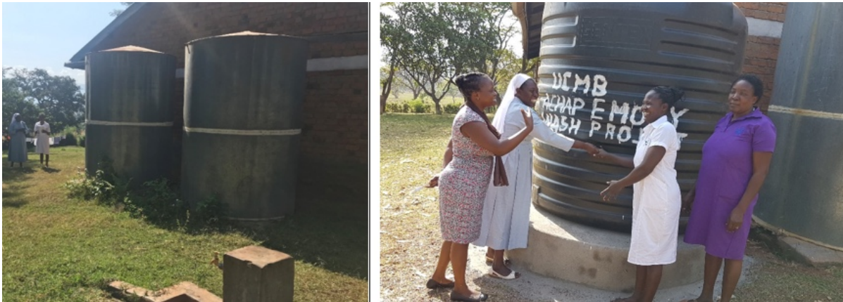
Above: Before and after photos of water storage tanks at a UCMB health center (Photo Credit: Monicah Luwedde/ UCMB)
