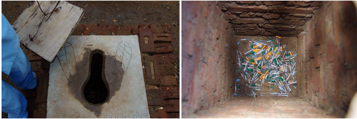
311 312 A B 313 Fig. 3 Low-cost sharps pit modified from pit latrine design A.) Surface of the pit as covered with a 314 repurposed precast pit latrine slab and drop-hole cover. B.) Inside the unlined pit showing segregation 315 of sharps.
