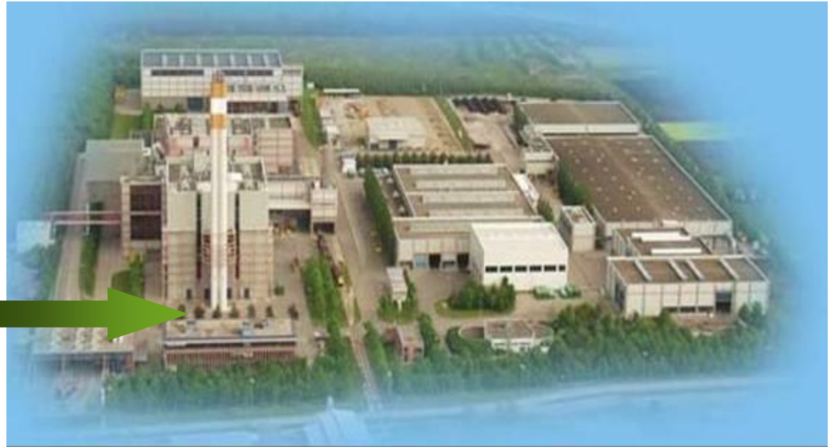
Waste treatment center, Augsburg with household waste and special waste incinerator.
