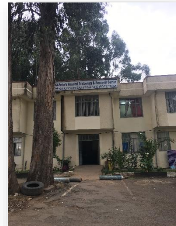
Figure 2 Departments at St Peter’s Hospital, yet to be renovated
