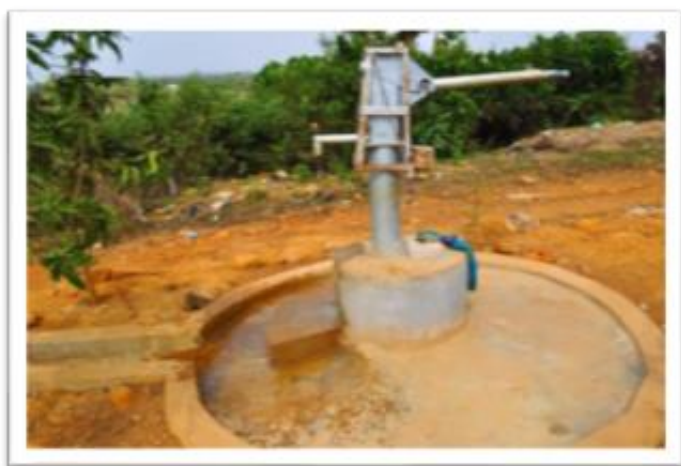
Figure 1. Close-up of the dug well with a hand pump
