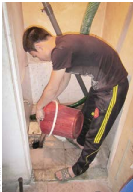
Photo 1: Adding water to facilitate extraction of settled sludge at the bottom of the tank within the truck.
