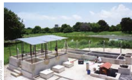
Photo 1: Faecal sludge dewatering research facility at the University of Dar es Salaam in Tanzania.
