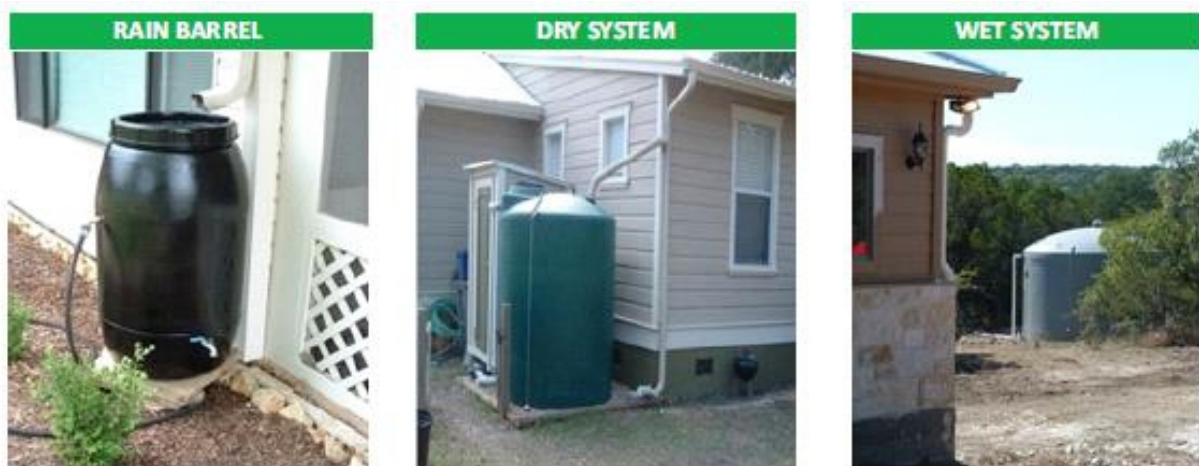
Figure 4: Diagram for different method to collect rainwater, adapted from Federal Ministry of Health, Nigeria. 2022. National Guidelines for Water, Sanitation and Hygiene in HCFs in Nigeria
